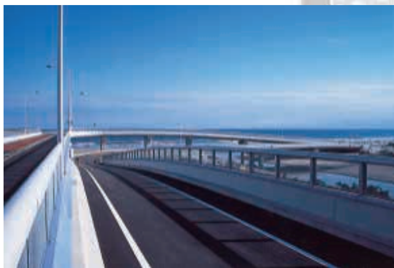
東金九十九里有料道路が開通(1998) Opening of the Togane Kujukuri Toll Road
