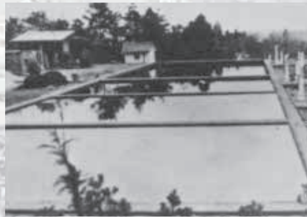
雄蛇ヶ池浄水場完成(1957) Completed Ojagaike Water Treatment Plant
