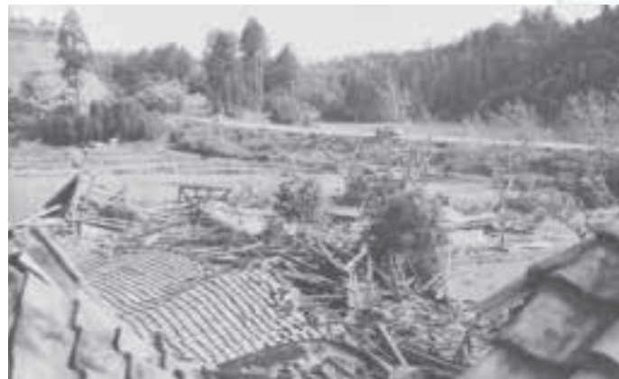
悪夢の一夜、台風34号の被害(1967) Damage from the nightmarish night when Typhoon 34 struck
